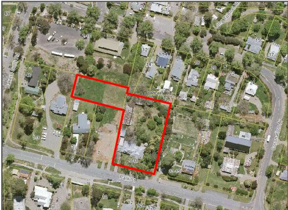
Figure 2: Subject land and surrounds.
