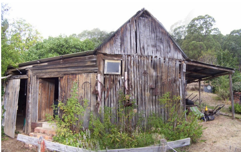
Slab Cottage, Dairy & Cellar
