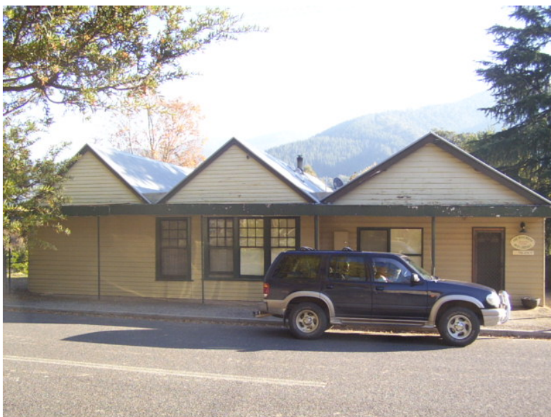
General Store, former
