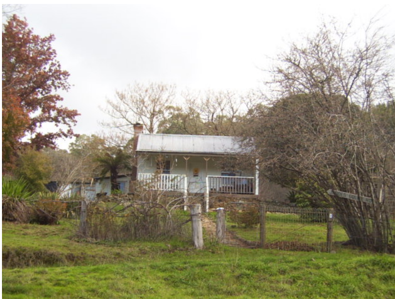
Cottage; 2 Jagoes Gully Road, WANDILIGONG
