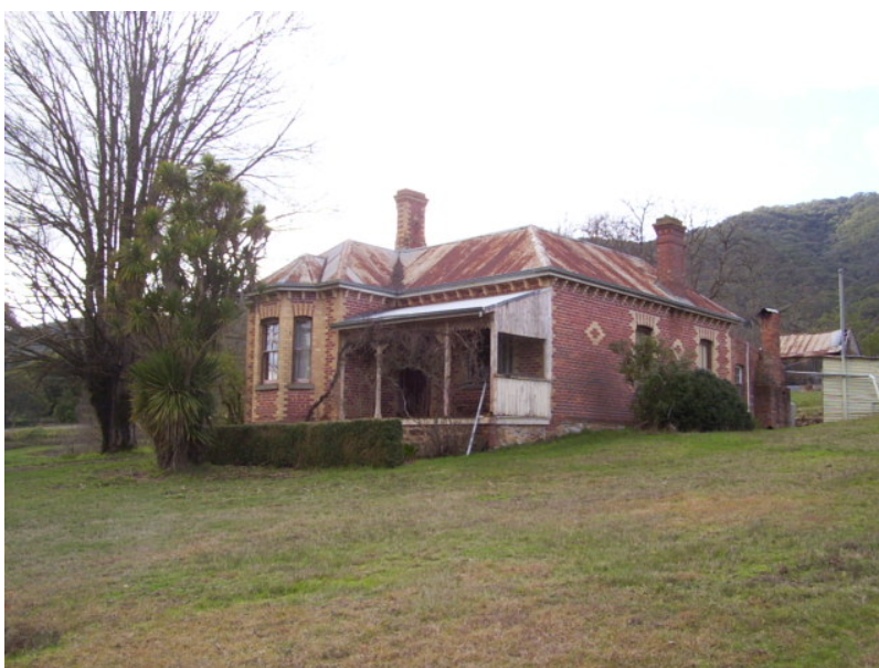
House; Peabody Road, WANDILIGONG
