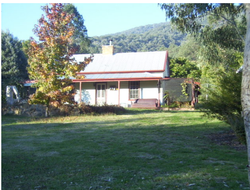
Police Residence, former
