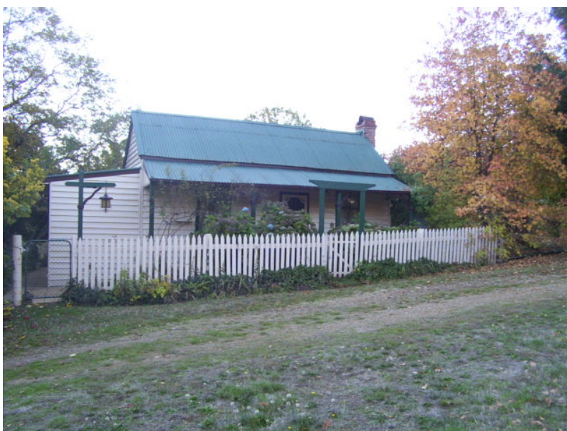
Cottage; Smithy Road, WANDILIGONG
