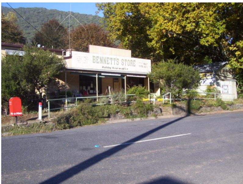
General Store, former
