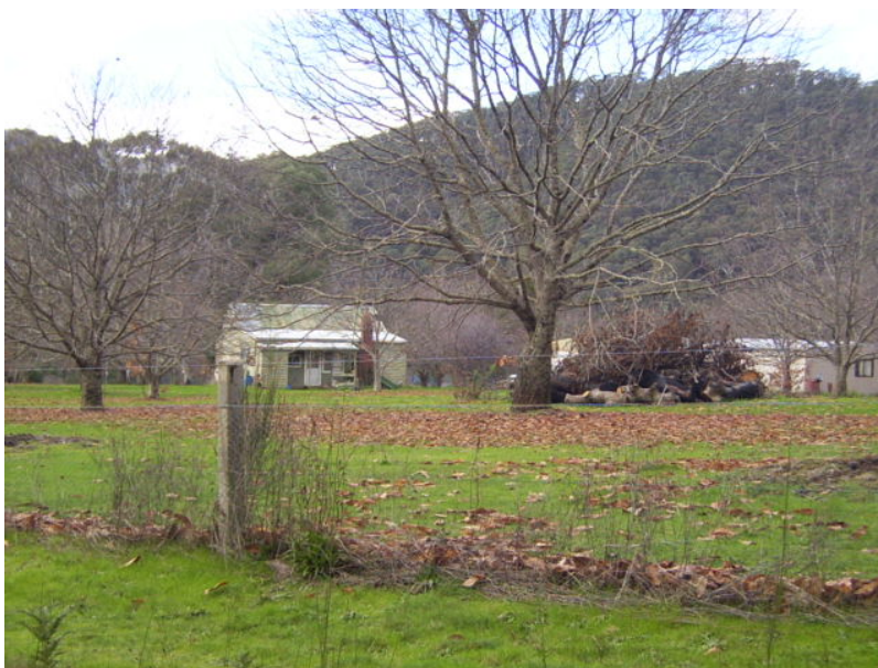
Cottage; 37 Jagoes Gully Road, WANDILIGONG
