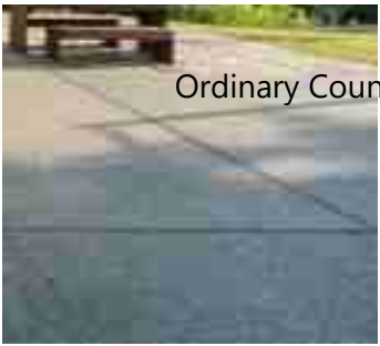
[P1] Coloured exposed aggregate insitu concrete with local aggregate and sawcut joints
