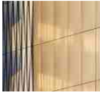
[SH1] Shelter ceiling cladding material 1 = gold-coloured anodised aluminium sheeting with lazercut lettering (content to be advised) [SH2]
