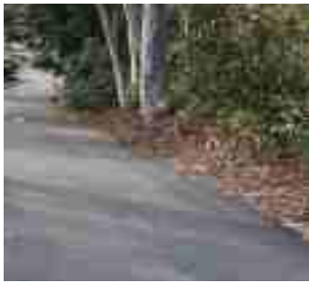
[P4] Asphalt road pavement without kerb and channel
