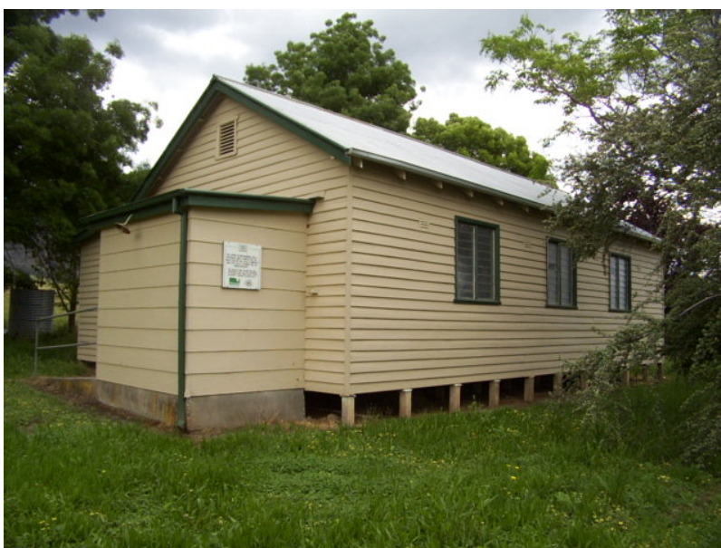
Upper Gundowring Hall
