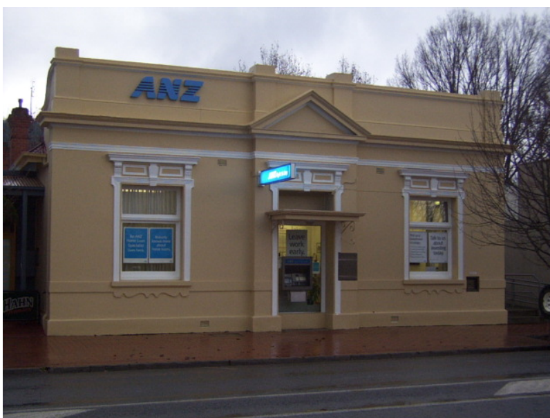
ANZ Bank Building
