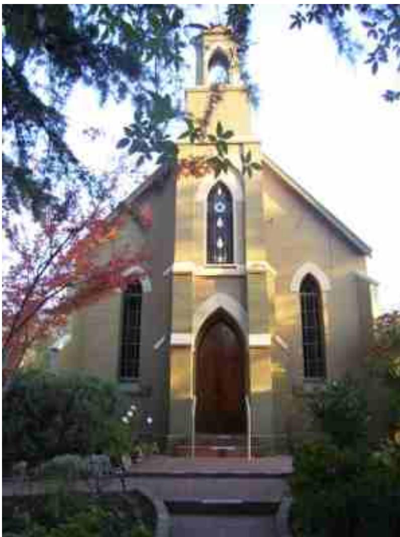
St Andrews Church, former
