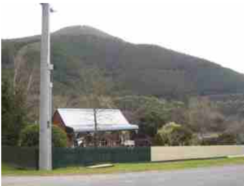
Blacksmith's Shop, former
