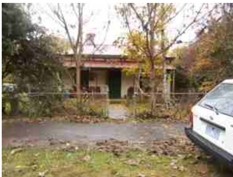
Police House, former
