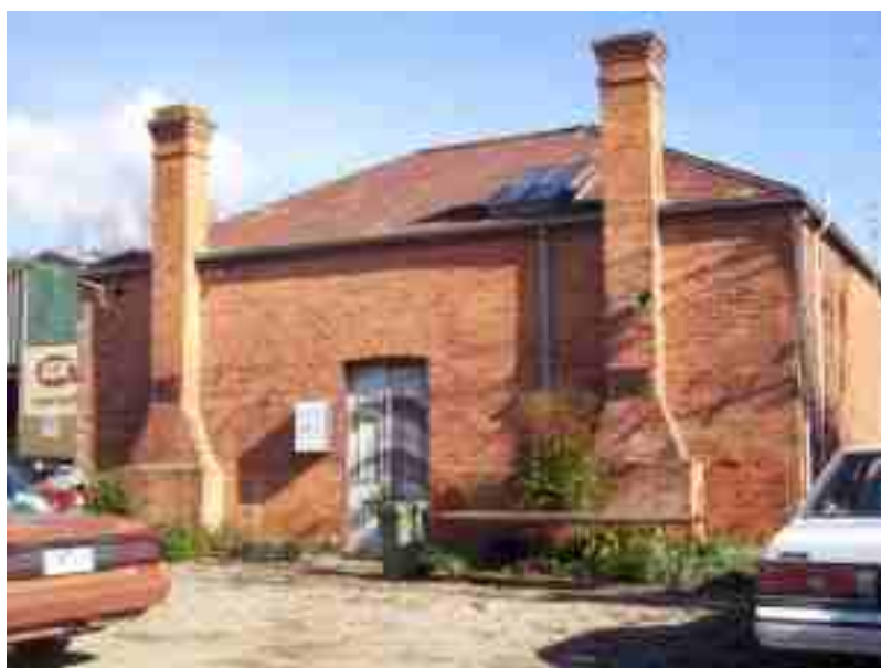
Supper Room, Victoria Hall, former
