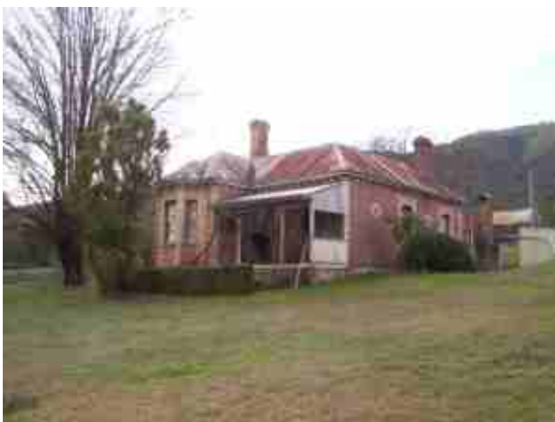
House; Peabody Road, WANDILIGONG
