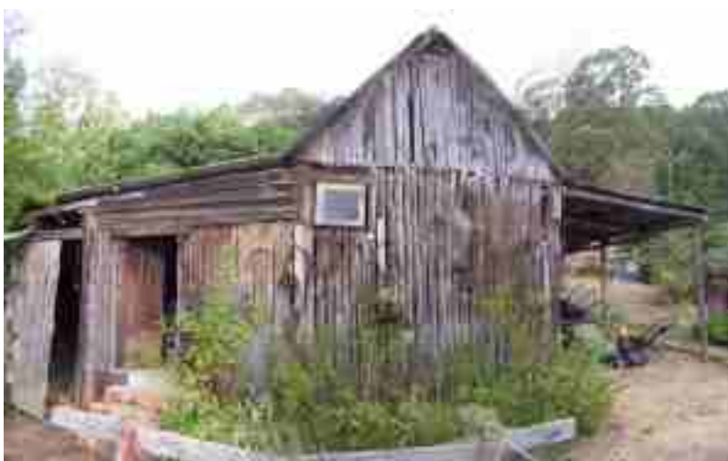
Slab Cottage, Dairy & Cellar
