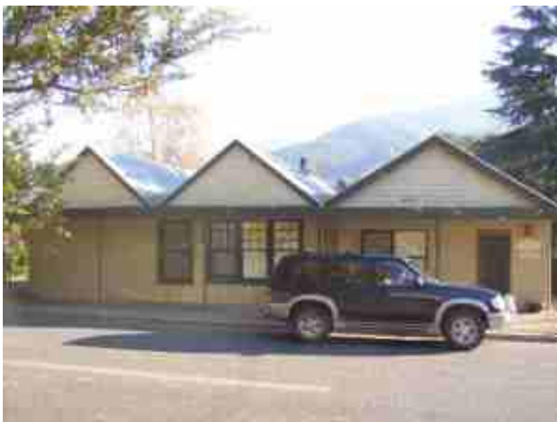
General Store, former
