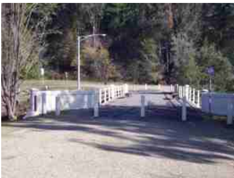
Old Porepukah Bridge
