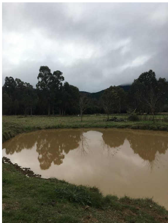
Figure 4: Dam to be removed
