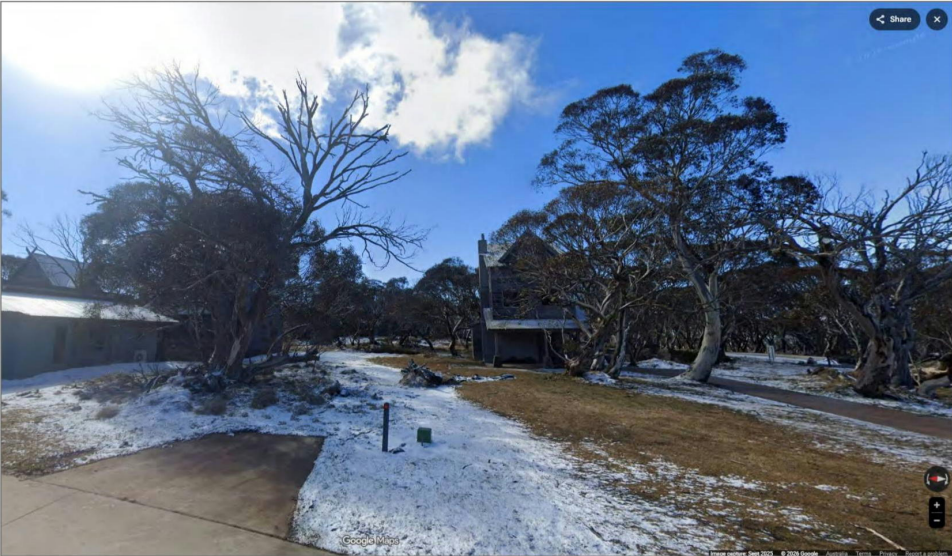
No. 8 (CENTRAL SNOW COVERED) & No. 6 (VACANT FOREGROUND RIGHT) & No. 4 (DWELLING BACK RIGHT) OF RONEY MACS TWIST - IMAGE FROM GOOGLE MAPS STREETVIEW, SEPTEMBER 2025
