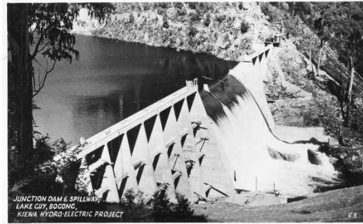
Junction Dam c1950 (photo © State Library of Victoria)
