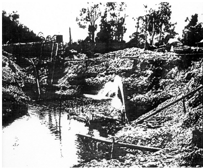
Hydraulic sluicing at Harrietville, c1900 (photo courtesy Harrietville Historical Society)
