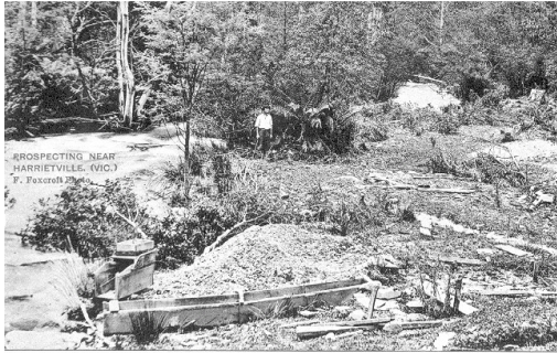
Small-scale alluvial mining at Harrietville, c1900 - note sluice-box and cradle in foreground (Foxcroft photo from postcard in R Kaufman collection)
