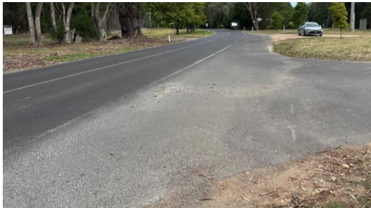
Figure 6.7: Recommendation 18 – Typical Pavement Marking Deterioration at Local Road Intersection
