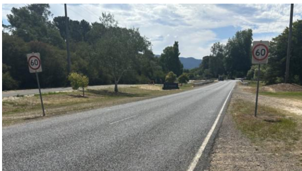
Figure 5.9: Back Porepukah Road – At 60 km/h Speed Limit Zone facing Porepukah
