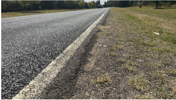
Figure 5.3: Back Porepukah Road – Typical Road Pavement Edge
