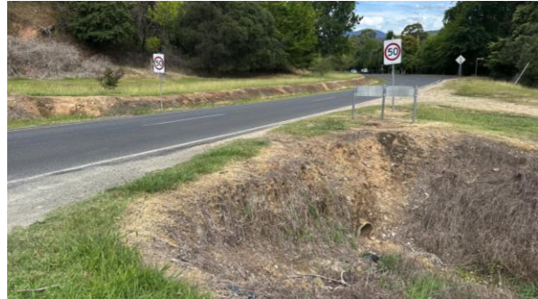
Figure 6.4: Recommendation 4e – Open Drainage Channel
