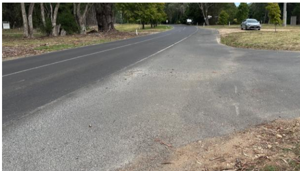
Figure 6.7: Recommendation 18 – Typical Pavement Marking Deterioration at Local Road Intersection
