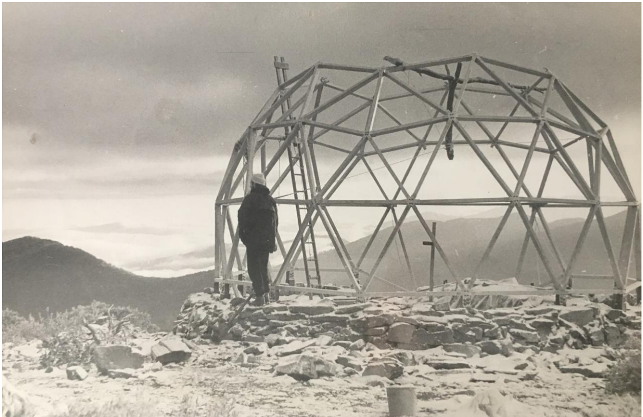
Circa 1965-66, during construction (Source: MUMC Facebook Group)
