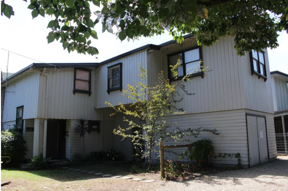
West elevation (Source: RBA, March 2024)
