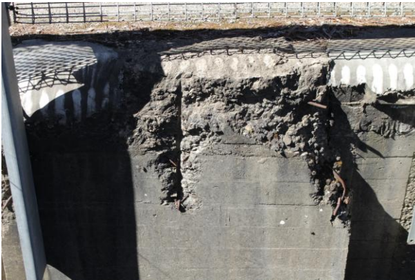
Germantown Concrete Bridge – detail of the pilster with exposed reinforcement, left, and remnant, dislodged panel from the balustrade, right (Source: RBA, March 2024)
