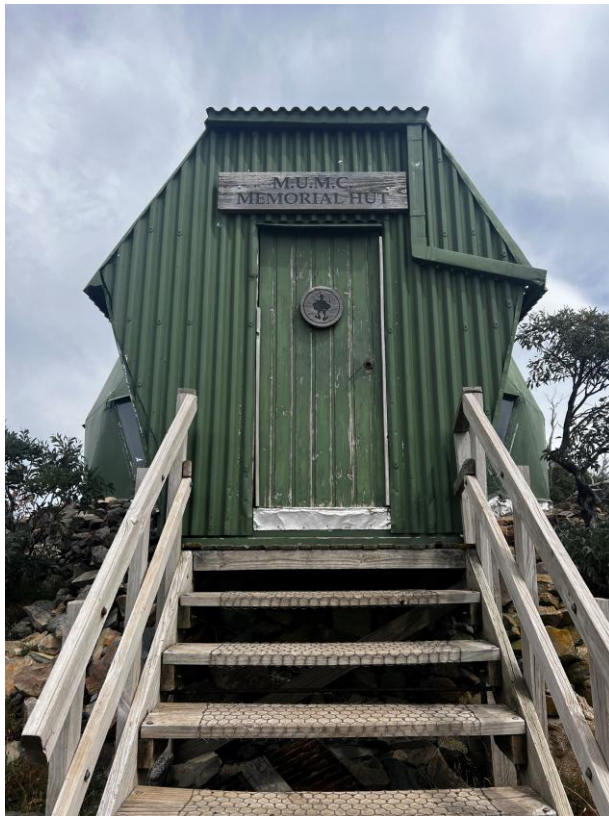
Entry/anteroom (Source: RBA, March 2024)
