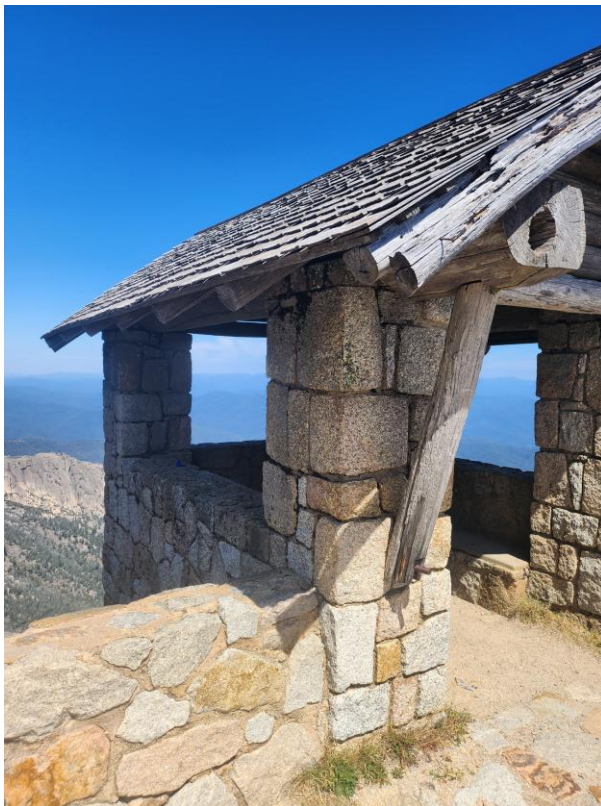
Side view and roof (Source: RBA, March 2024)
