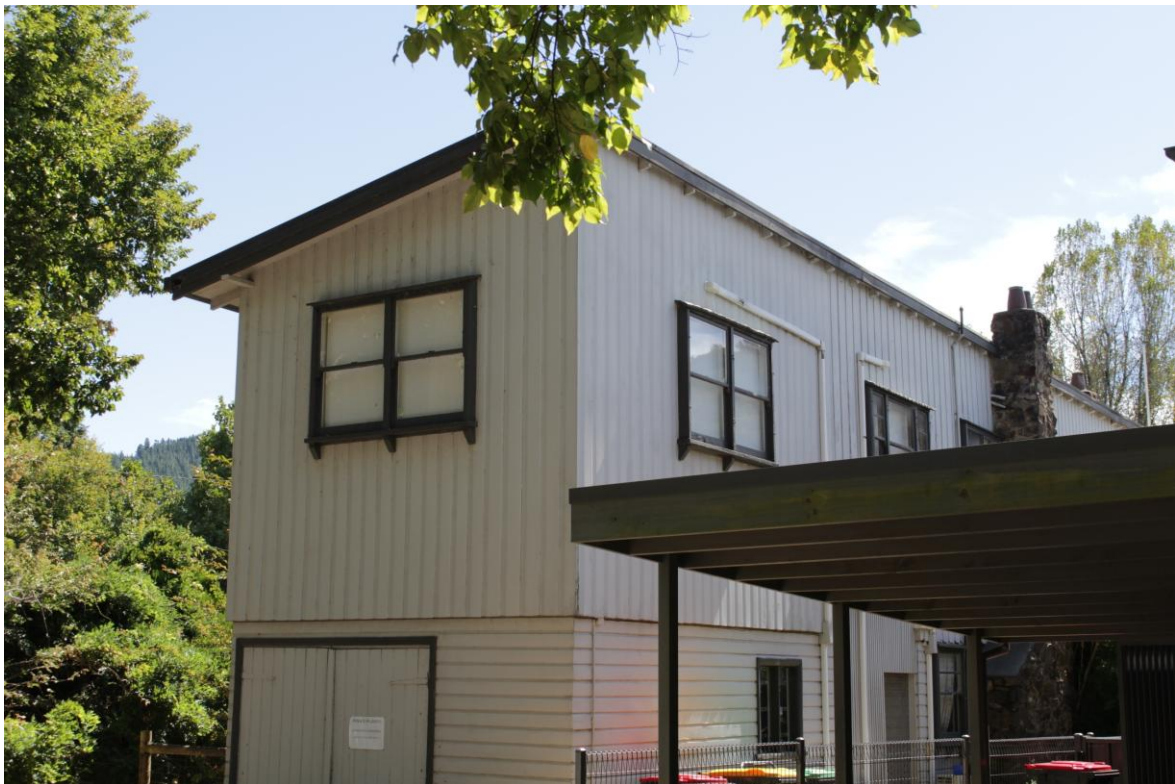
East elevation (Source: RBA, March 2024)
