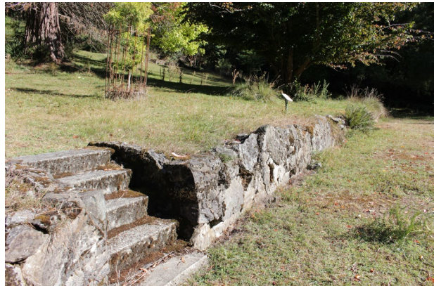
Retaining wall and stair
