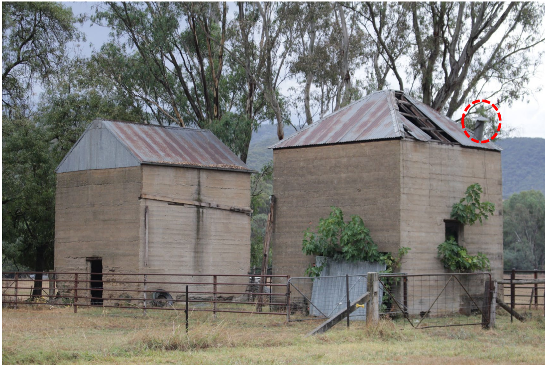
39 Briggs Lane – note the remnant flue to the front kiln (Source: RBA, March 2024)
