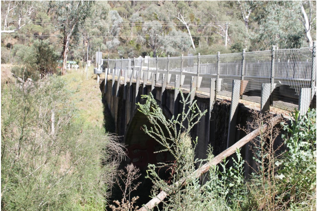
Germantown Bridge (Source: RBA, March 2024)
