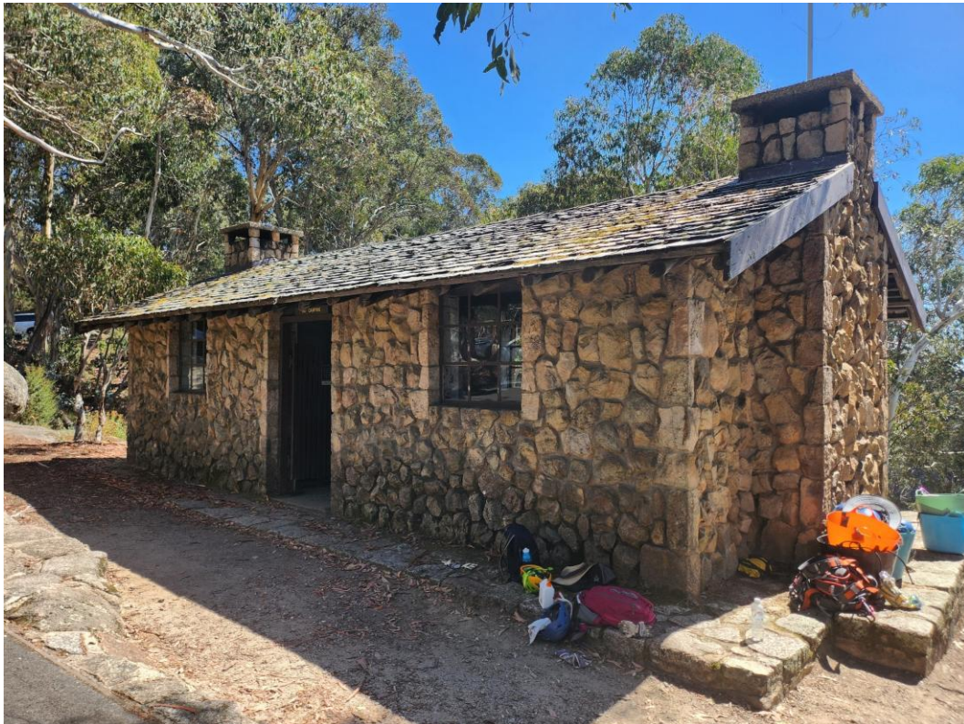
Echo Point Shelter Hut (Source: RBA, March 2024)
