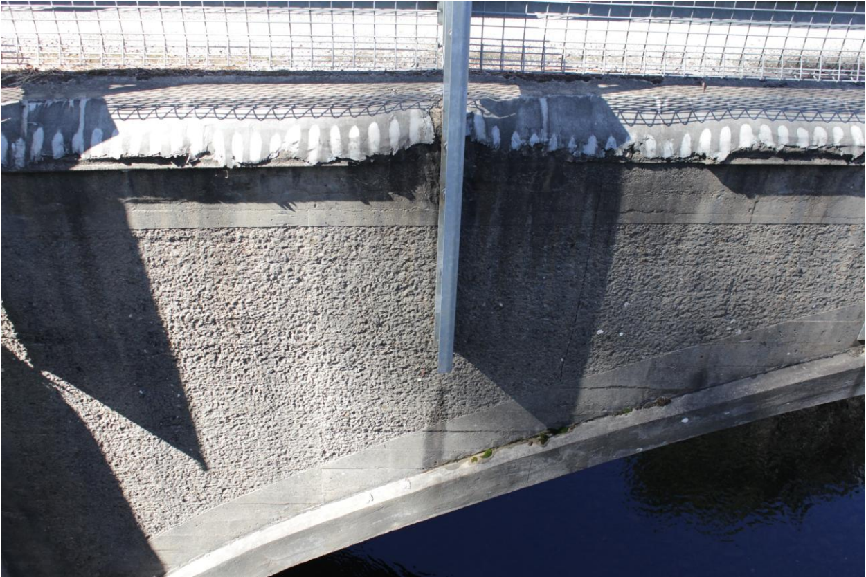
Germantown Concrete Bridge – detail of the spandrel showing contrasting finishes (Source: RBA, March 2024)
