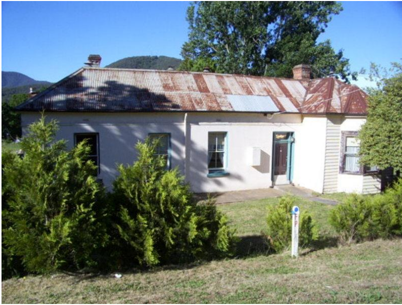
Façade in 2008 (Source: Hermes)
