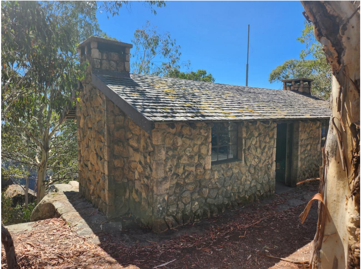
Echo Point Shelter Hut (Source: RBA, March 2024)
