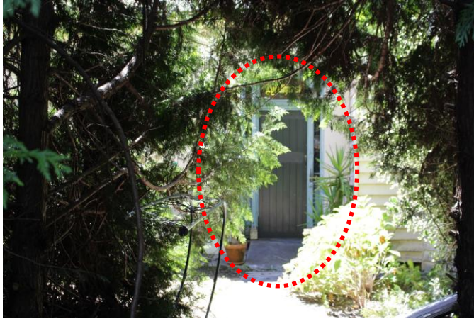
Former Lyndhurst Private Hospital, showing current front door (Source: RBA, March 2024)
