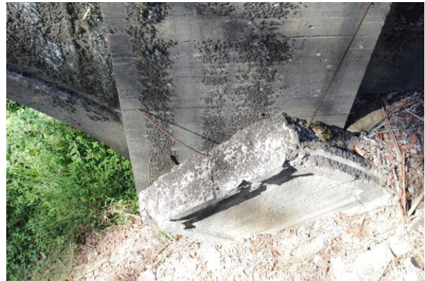
Germantown Concrete Bridge – detail of the pilster with exposed reinforcement, left, and remnant, dislodged panel from the balustrade, right (Source: RBA, March 2024)
