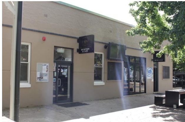
Late 20 th century addition, corner of Barnard Street
