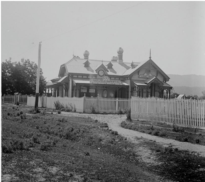
Circa 1900, Myrtleford Post Office and Court House (John Henry Harvey), with the later memorial square area on right (Source: SLV, H86.76/5)
