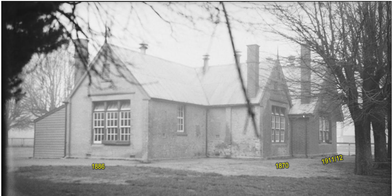
Photograph of State School No. 955 (Former) showing north (right) and east (left) elevations. Undated but likely late interwar period. Note the brick for the 1870 and 1886 wings appears to have a thin applied finish, possibly a lime or brick wash. (Source: Public Works Department, VPRS 10516/P0001, PROV)
