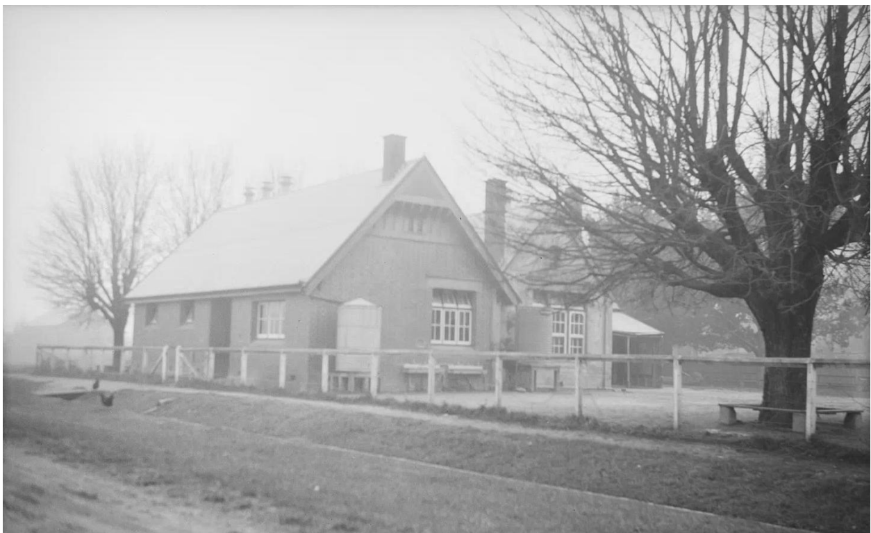
South elevation, from Elgin Street. (Source: Public Works Department, VPRS 10516/P0001)
