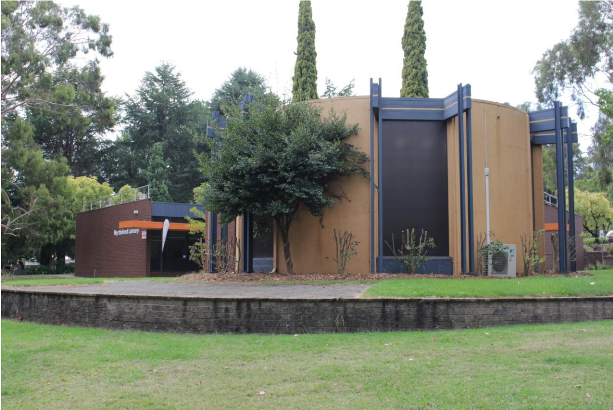
Former council chambers/'drum', viewed from the landscaped area at the southern tip of the triangular holding. (Source: RBA, March 2024)
