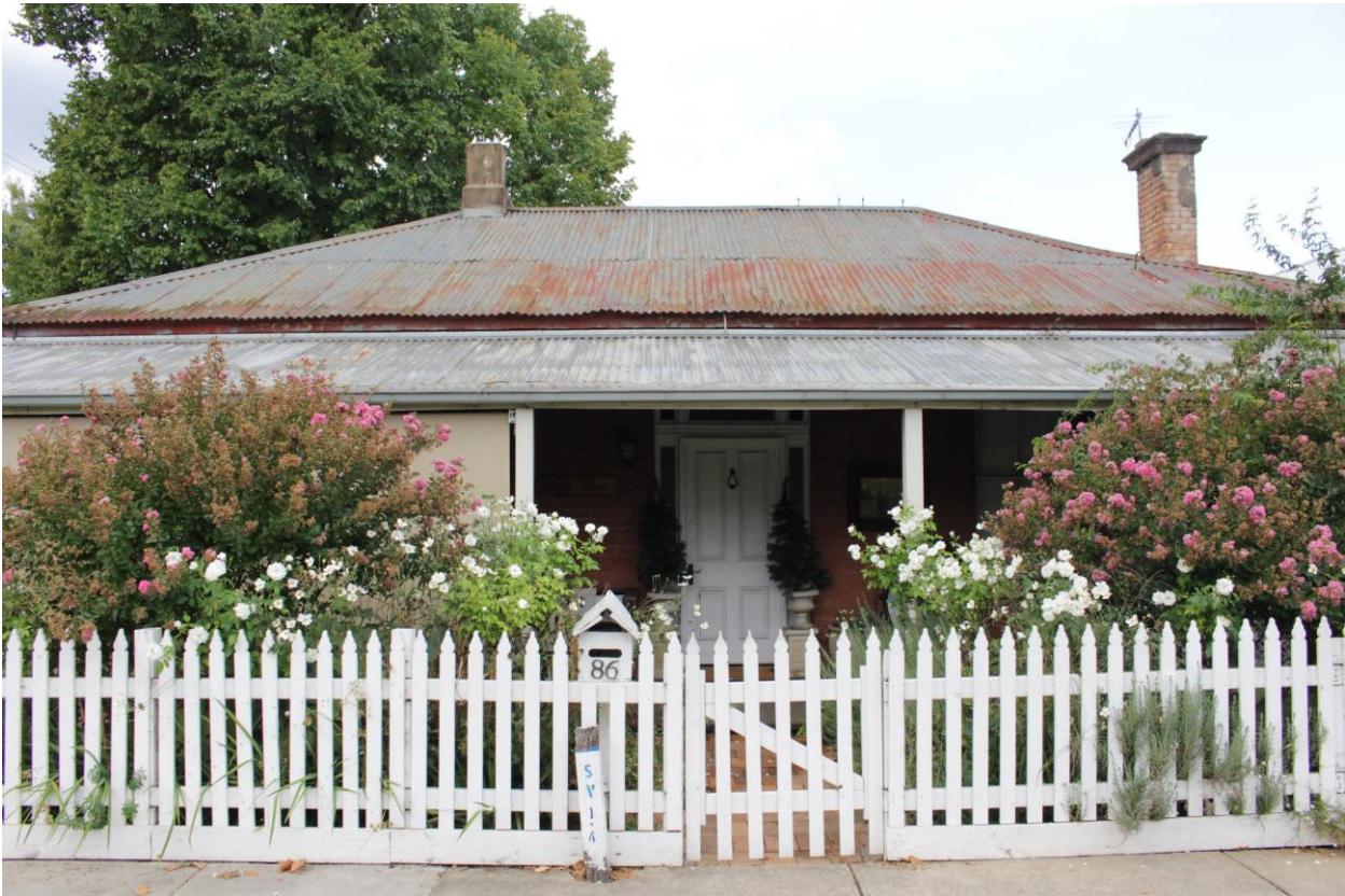
Mathieson/Rothery Residence, Myrtle Street. (Source: RBA, March 2024)
