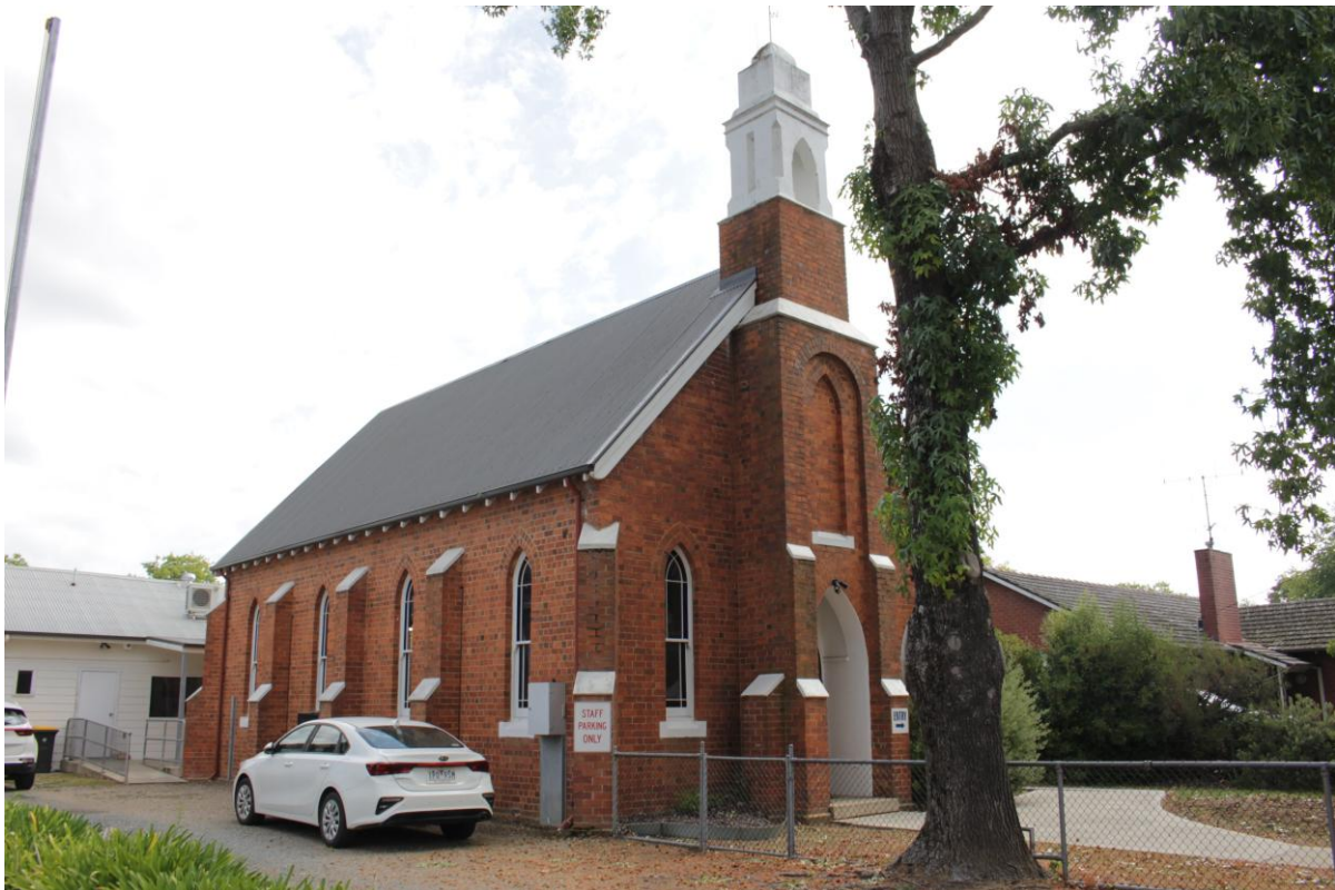
St Andrew's Church – façade and east elevation, from Smith Street. (Source: RBA, March 2024)
