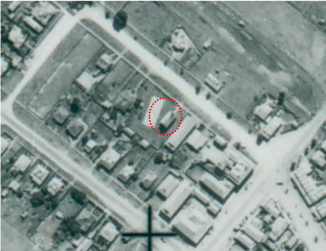
Aerial photograph of St Andrew's (red arrow), dated 1948. The liquidambar trees to the front were not established (or had not been planted) but there was a tennis court (since developed) to the north of the church. (Source: Mapsheet Photography, Bright, Run 4, Frame 145, Geoscience )
