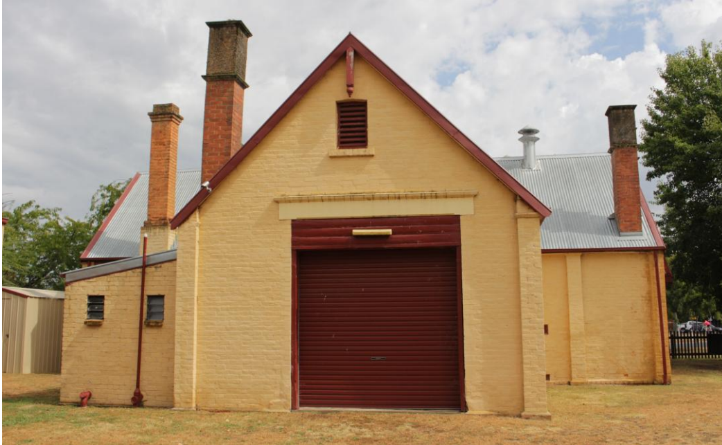
Façade (east elevation) of the 1886 wing. (Source: RBA, March 2024)
