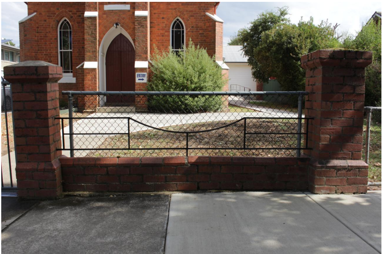
Section of the brick front fence, with metal railing, dating to 1937 (Source: RBA, March 2024)
