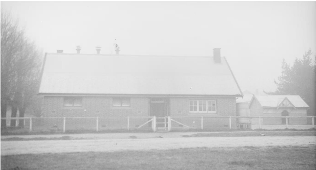
West elevation (Elgin Street), likely interwar period. The timber building right of frame may be the 1915 shelter shed. (Source: Public Works Department, VPRS 10516/P0001)
