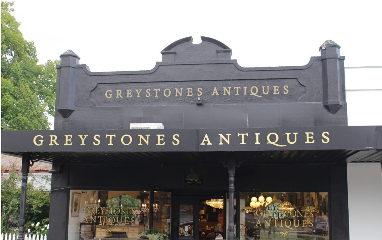
Pedimented parapet. (Source: RBA, March 2024)
