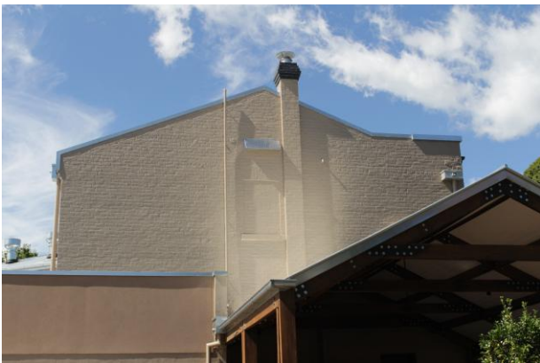
Gable end at west end
