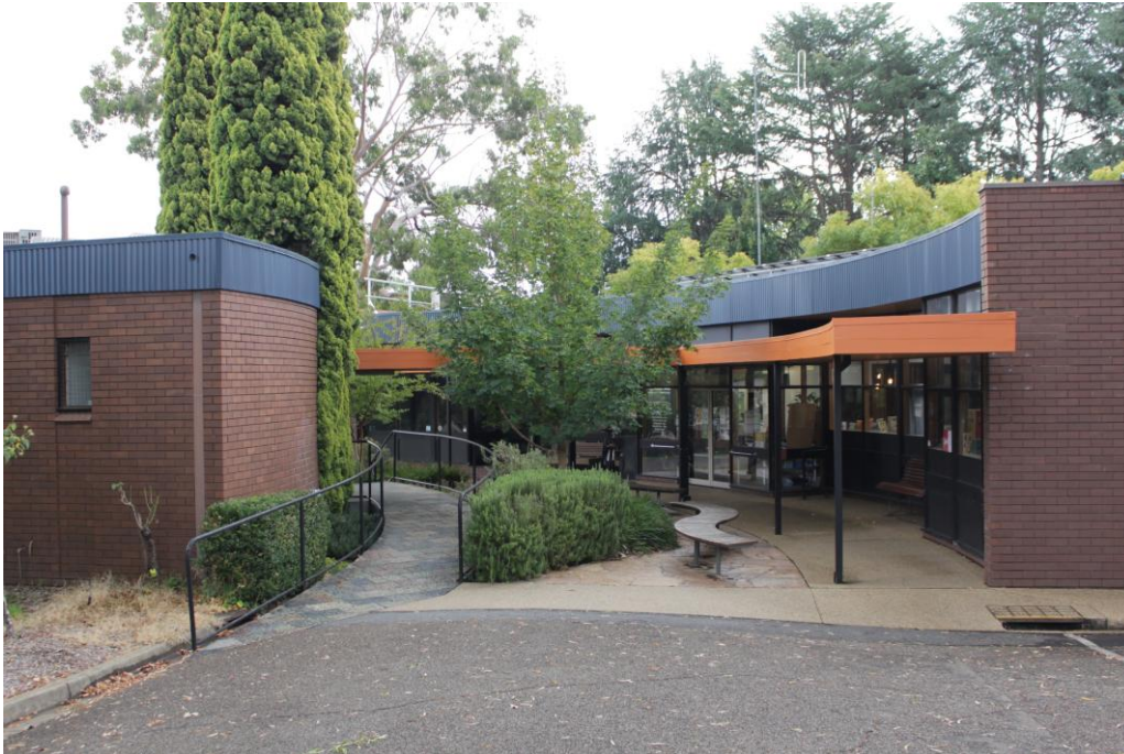
'Windowall' of the former municipal office's south elevation (right), from the east/Standish Avenue. (Source: RBA, March 2024)
