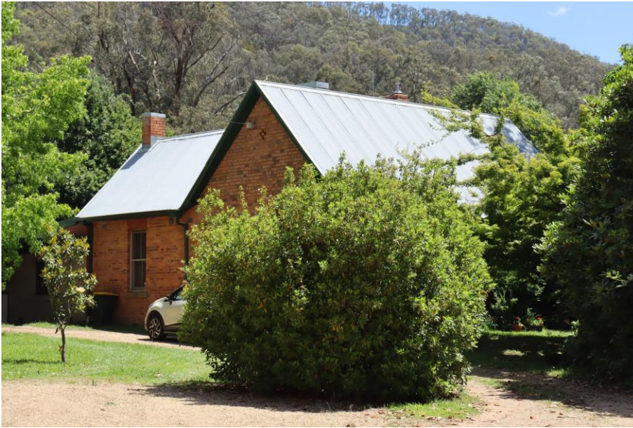
Parsonage, north-east part (Source: RBA, December 2024)
