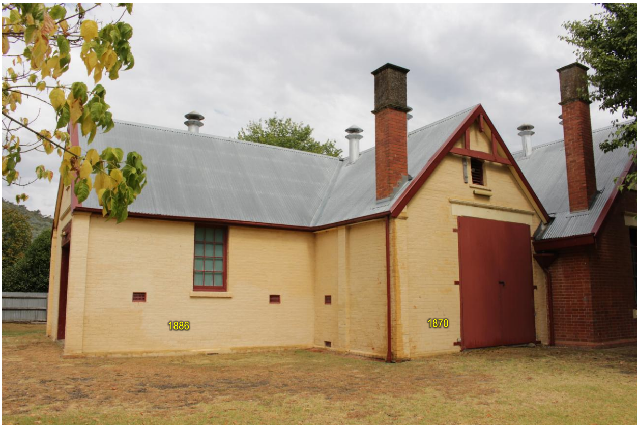
North elevation, 1870 wing (right) and 1886 addition (left). (Source: RBA, March 2024)
