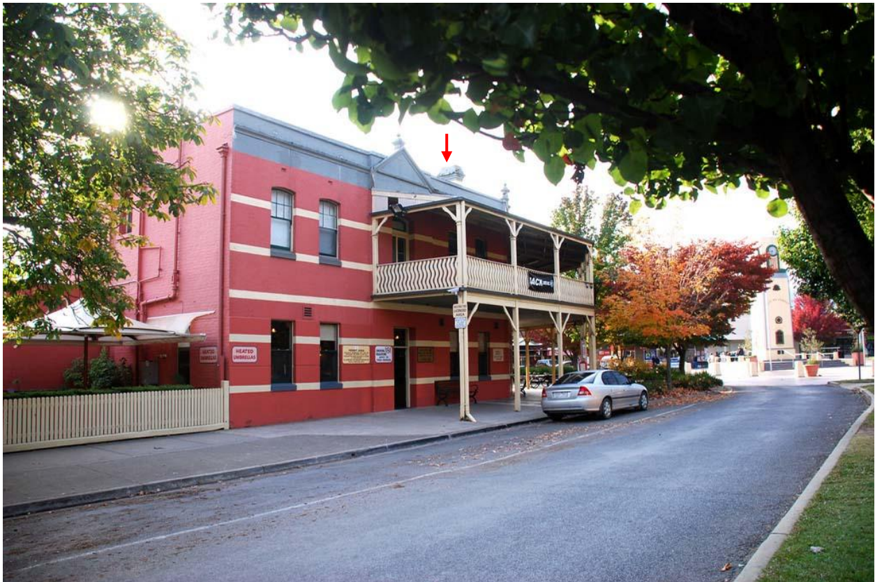
Circa 2008, showing original colour scheme in the paintwork Note the reinstated chimney cap (Source: Council)
