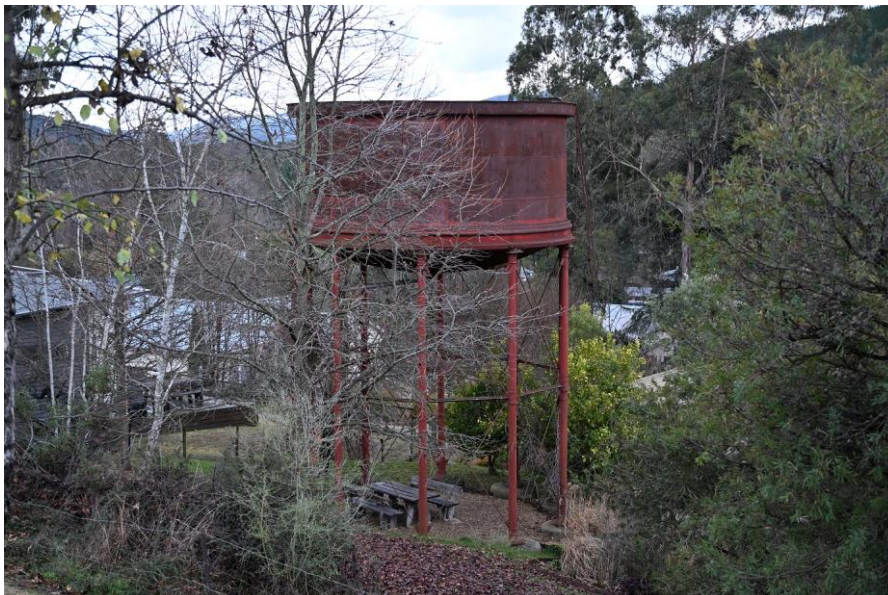
Water tower from south, from Rebecca Drive (Source: Council, June 2025)
