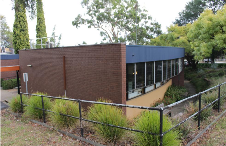
Former municipal offices, now library, from Standish Street, showing north (rear) and east (side) elevations. (Source: RBA, March 2024)
