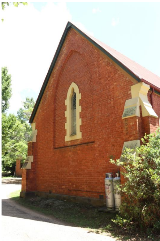
East elevation with blind niche
