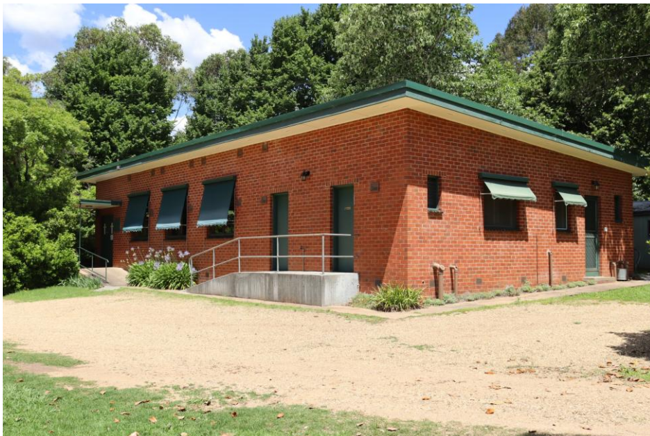
Sunday School/hall, north-west corner (Source: RBA, December 2024)
