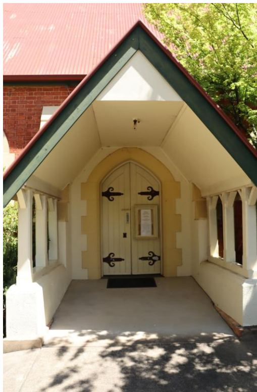
Entry porch (Source: RBA, December 2024)
