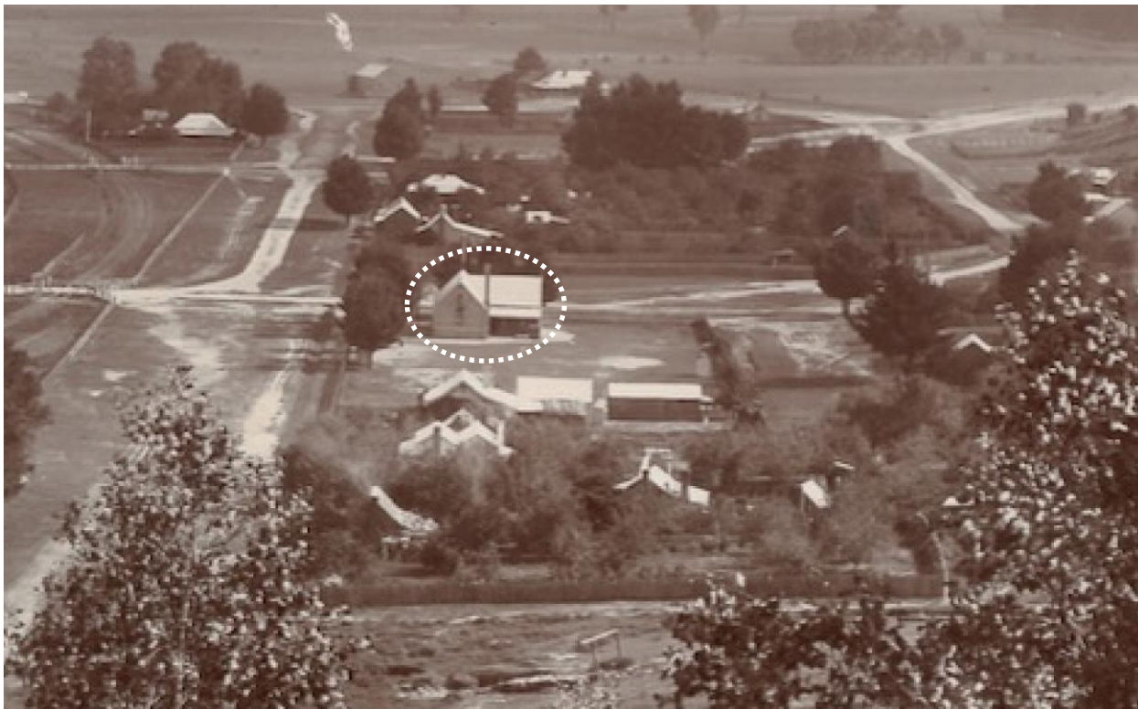
Extract from a photograph, dated 1890, showing the south elevations of the 1870/1878 and 1886 wings of Myrtleford State School No. 955 (circled). Note boundary plantings. (Source: Henry Van Heems/Vanheems, Myrtleford, RHSV Collection)
