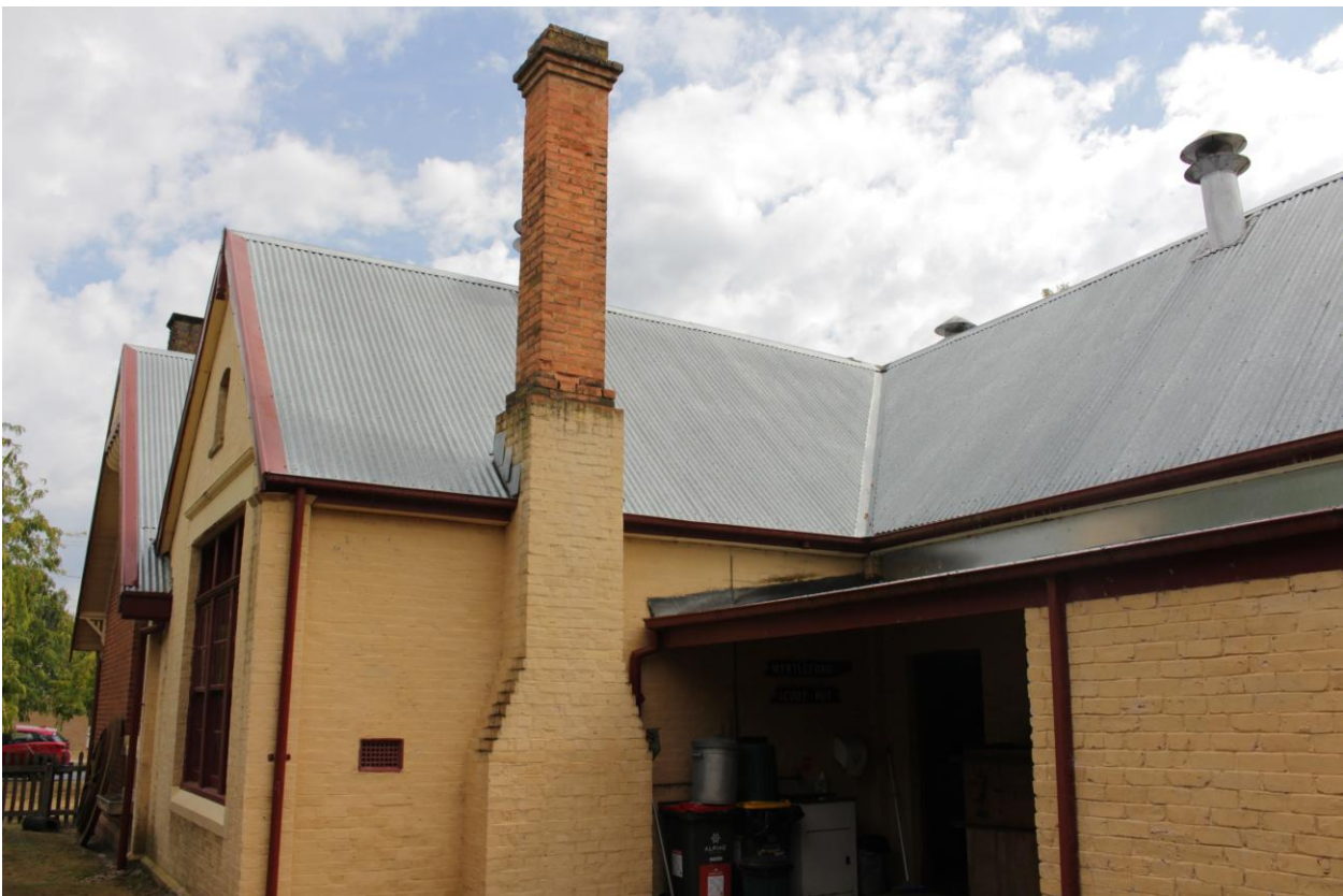
Close-up of the 1876 wing, facing west. (Source: RBA, March 2024)
