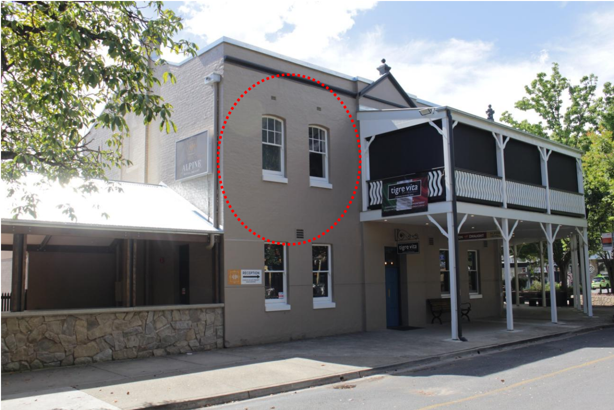
West end (Anderson Street), the underlying brickwork being faintly visible in the area highlighted (Source: RBA, March 2024)
