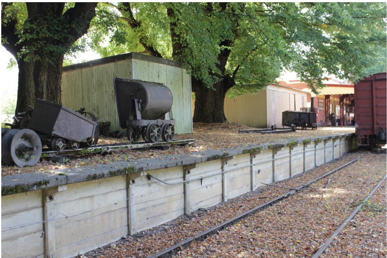
Platform, west end, with an early shed (foreground), large late 20 th shed (background), and English elms (Source: RBA, March 2024)
