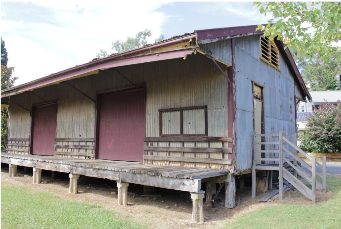
Goods shed, north-west corner (Source: RBA, March 2024)
