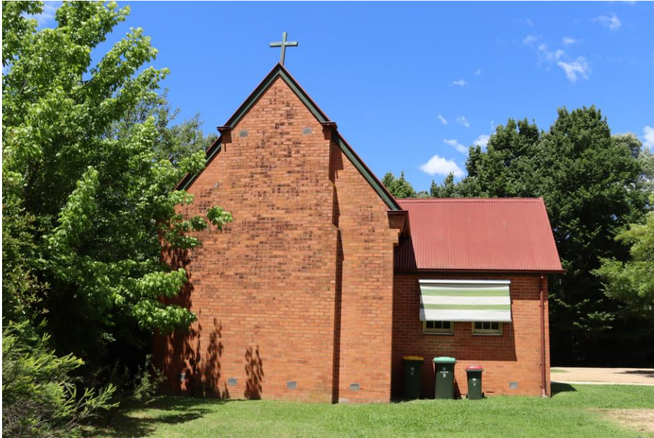
West elevation, showing 1950s completion – sanctuary (left) and vestry (right) (Source: RBA, December 2024)
