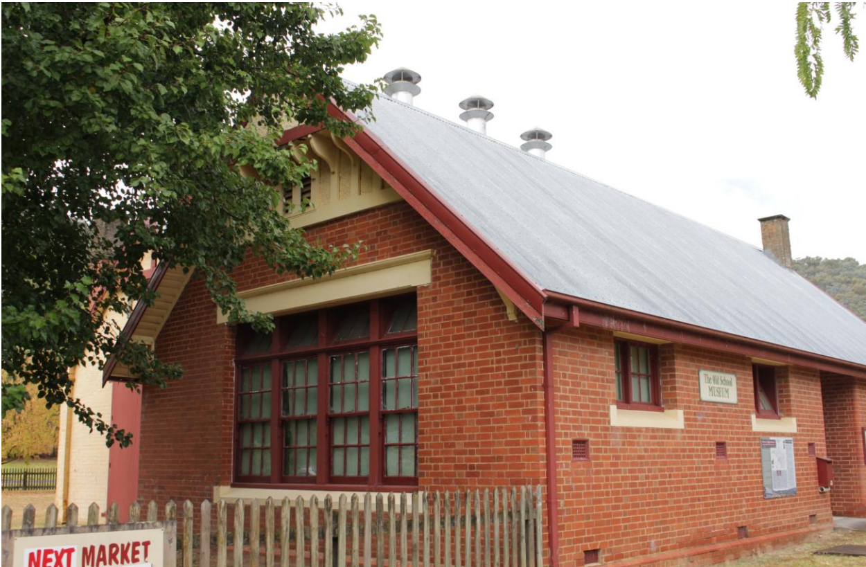
North elevation. (Source: RBA, March 2024)
