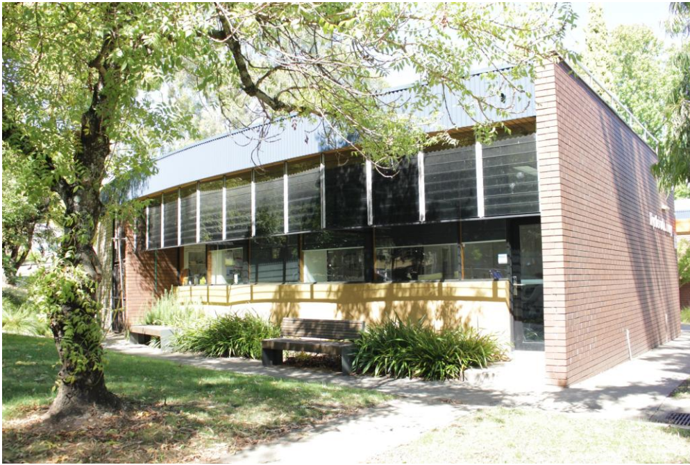
Rear elevation of the northern block, west bay. (Source: RBA, March 2024)
