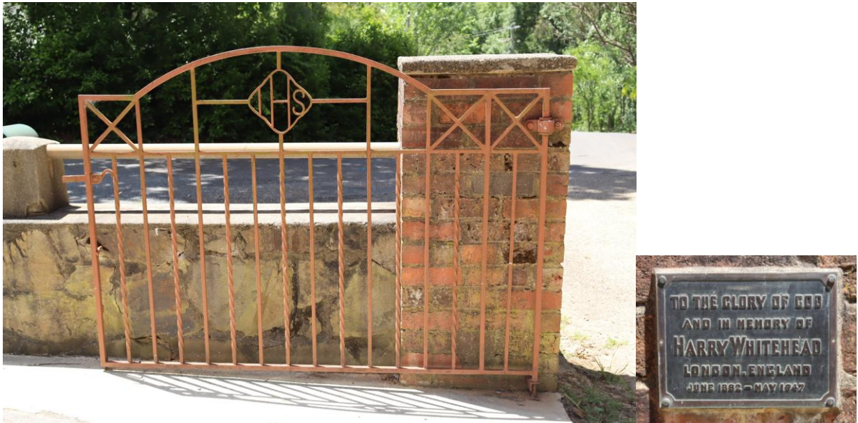
Front fence and plaque (Source: RBA, December 2024)
