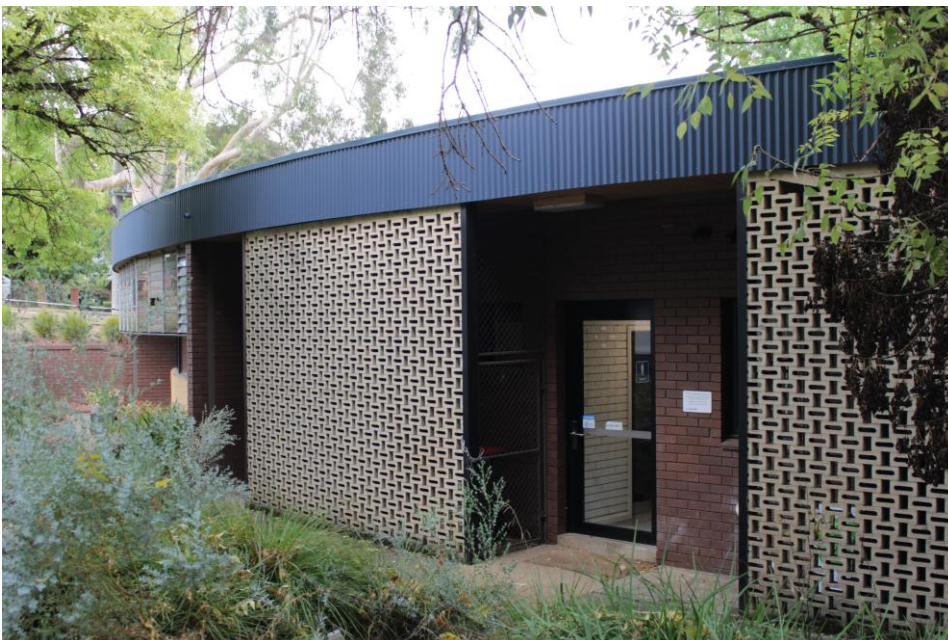
Central bay of the curved rear elevation of the northern block from the rear. (Source: RBA, March 2024)
