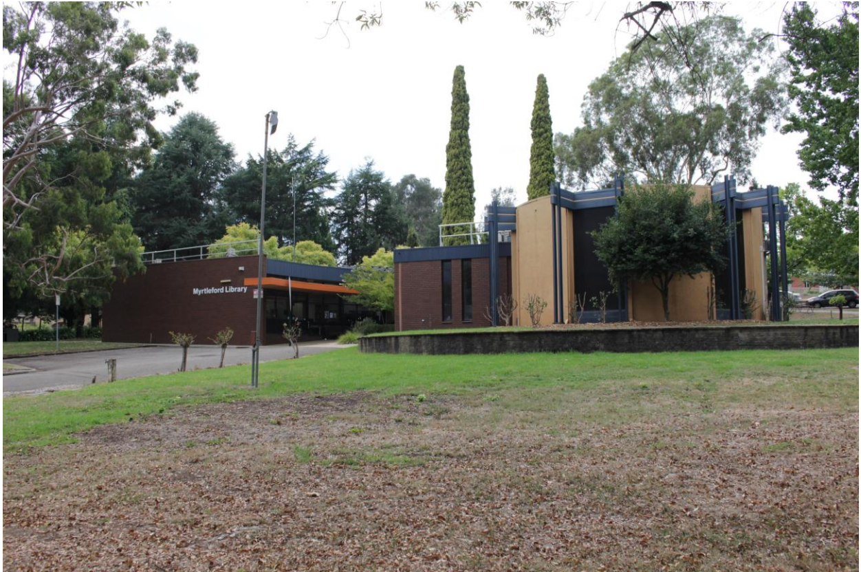
Site from the west/O'Donnell Avenue (Source: RBA, March 2024)
