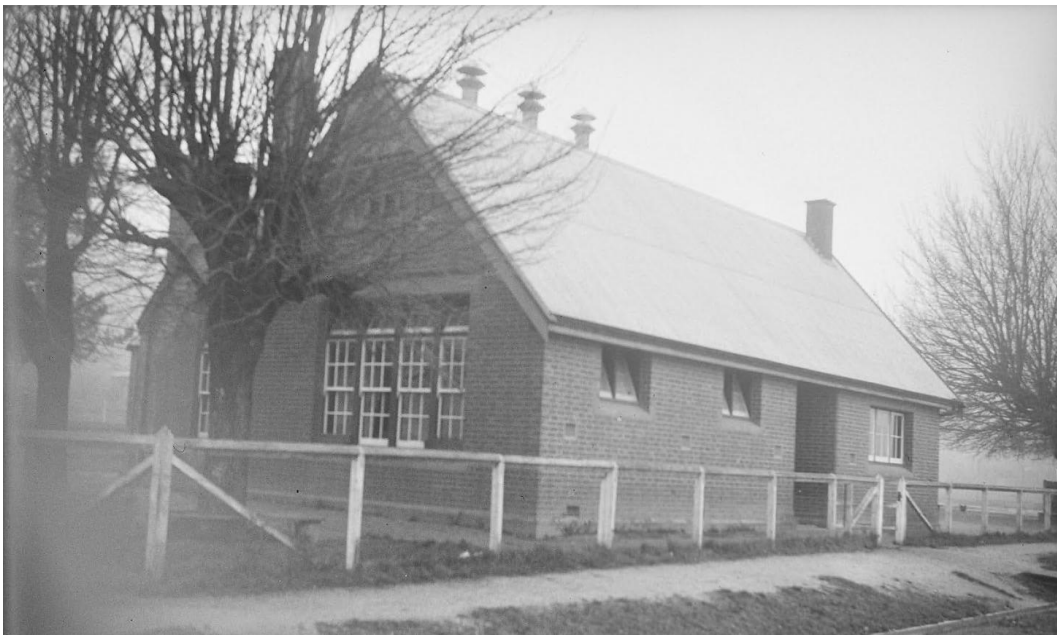
North (left) elevation, with the western (right) façade also shown, likely interwar period. (Source: Public Works Department, VPRS 10516/P0001, PROV)
