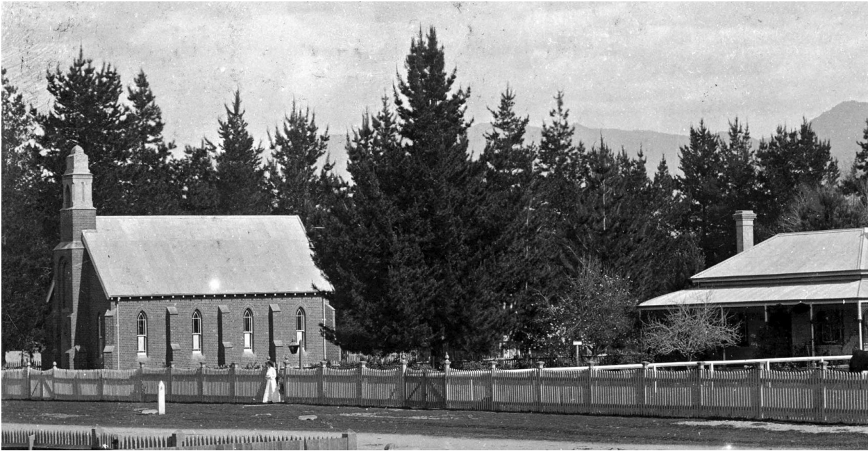
St Andrew's Church , circa 1905, from the north side of Smith Street. The façade and west elevation are shown. Note the original timber fence. None of the plantings captured survive. (Source: courtesy of the Myrtleford & District Historical Society)
