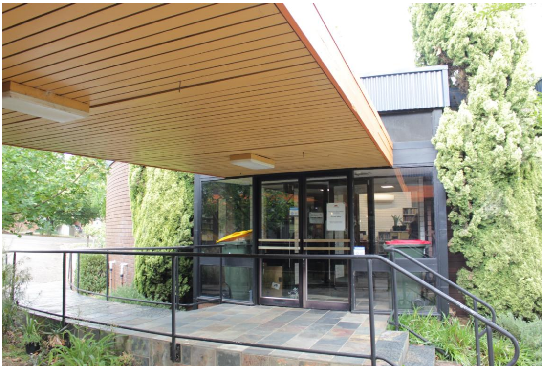
Entrance to the crescent-shaped porch/foyer (quadrant wing), former council chambers. The ramp is an addition. (Source: RBA, March 2024)
